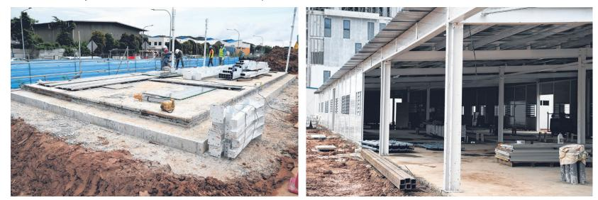
After land at the site is excavated and prepared, a concrete foundation is laid. Steel columns and beams are put up, forming the structure of the dormitory block. To speed up the process of construction, prefabricated steel beams that are manufactured offsite and which can be quickly assembled at the site are used.
