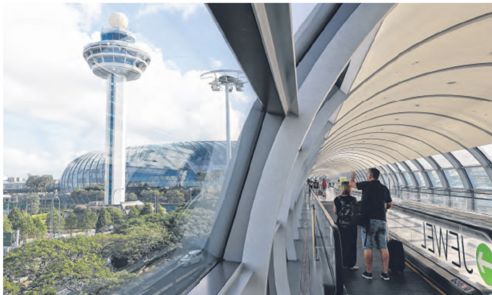
Located where an open-air carpark used to be, Jewel Changi Airport is a high-value, multi-functional commercial asset averaging a footfall count of 300,000 a day. Its unveiling is a demonstration of continual efforts to ensure that Changi Airport remains a leading international air hub, says the writer. ST FILE PHOTO
